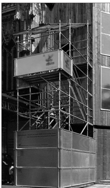
◀ Stairway tower (Layher interim stairway, max. load 5 kN/m 2 ) with Protect covering.
